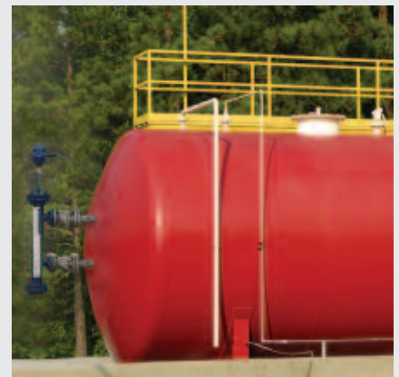
Fuel Oil Storage
